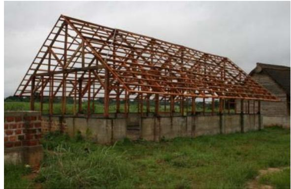
**19 Practical 1.** Finished the entire timber upper structure including vertical stands, window frames and veranda overhang (↑).
